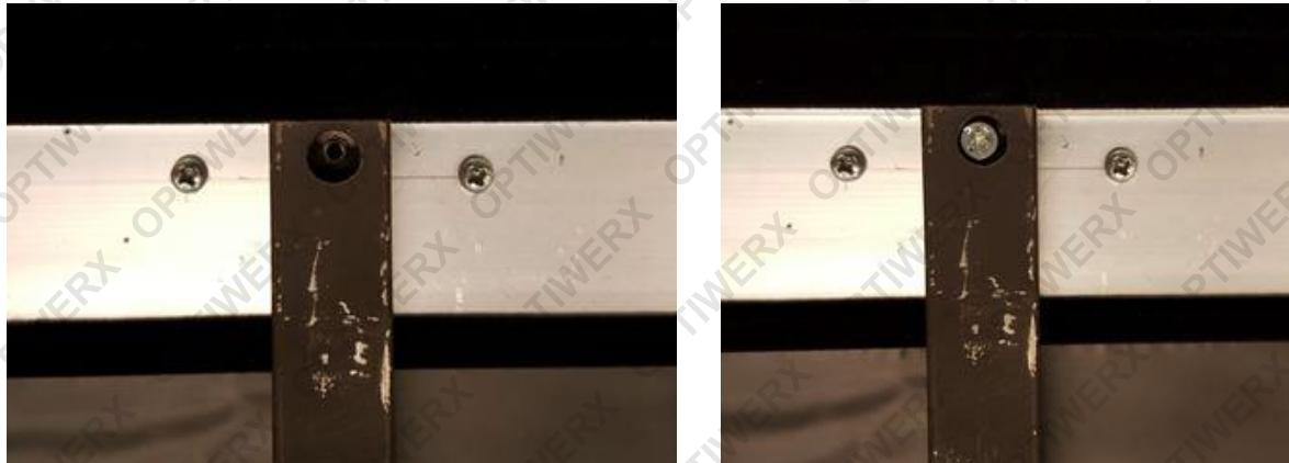
13. Using the spring tool provided, continue installing the springs along the bottom and top rail of the screen.
